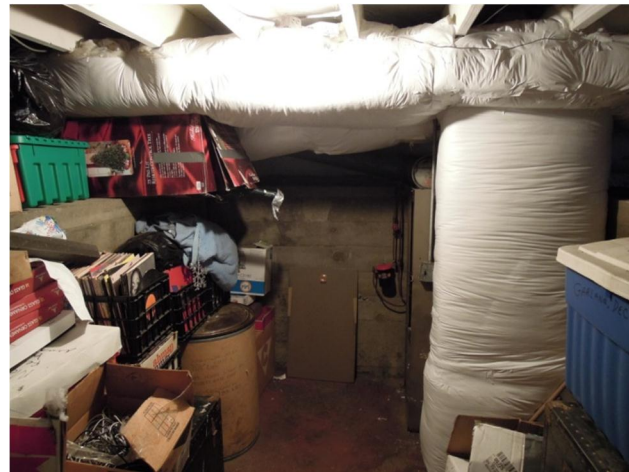
This client now has a completely sealed and insulated duct system. Her heat will no longer be seeping out into the unconditioned basement.
