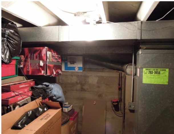
This client now has a completely sealed and insulated duct system. Her heat will no longer be seeping out into the unconditioned basement.
