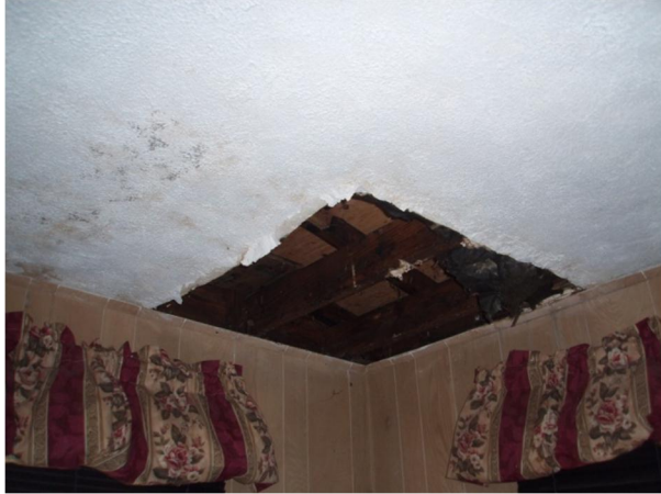
This client no longer has water-damaged ceiling (caused by major roof leak) in her bedroom which had a 3'x3' opening directly into the attic.
