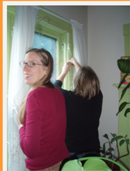
CEP Volunteers weatherizing a client's window with an internally-mounted, reusable storm window kit.
